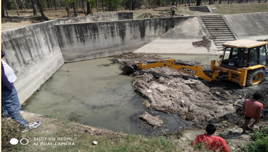
Clearing debris of Kachnapur Syphon of WMC
