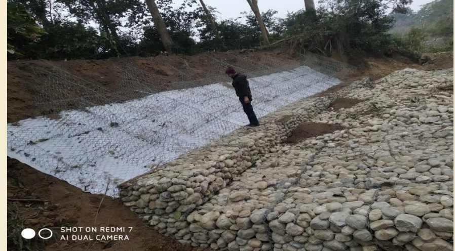
Carried Canal protection works at WMC
