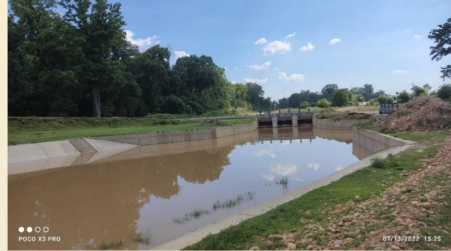
Desilting basin with Escape at Ch.0+500
