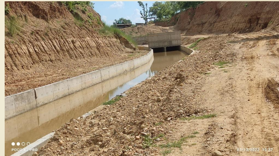
Box Barrel Canal at Ch 3+000
