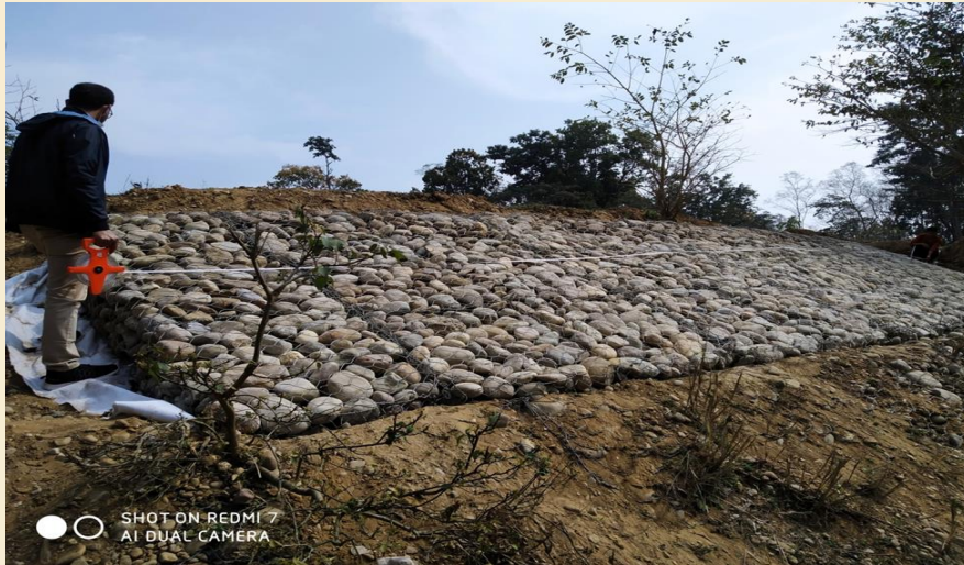
Taking Measurement of gabion slope protection works
