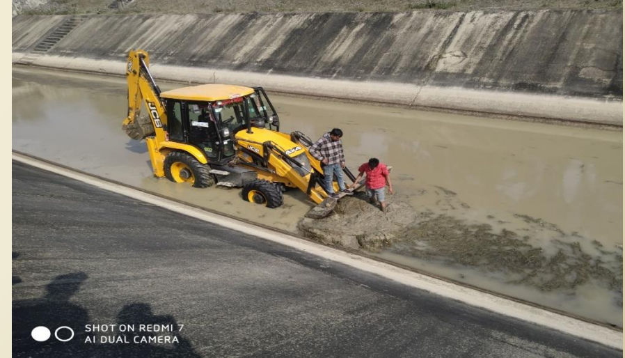
Clearing WMC for optimization of water delivery
